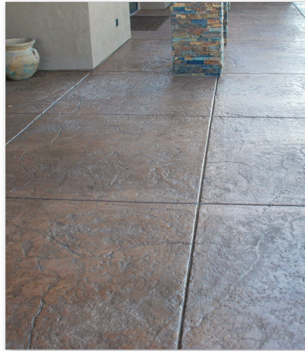
Fractured Earth embossing skin CHROMIX® ML Admixtures for Color-Conditioned® Concrete – Summer Beige LITHOCHROME® Antiquing Release – Walnut
